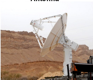
L/S/C Band Telemetry Tracking Antenna
