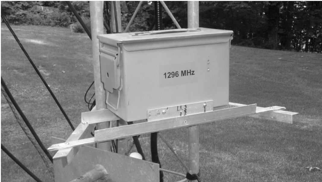
Figure 6 - RIG ATTACHED TO TOWER
