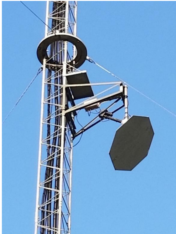
Figure 5. Flyswatter reflector with elevation/tilt control.
