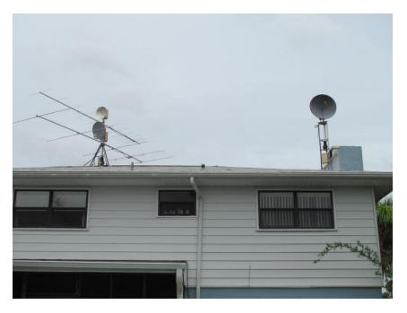
5760 MHz 7W to DSS dish @ 28ft 10368 MHz 7W to 3ft dish @ 30 ft All equipment is antenna mounted
