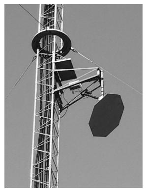
Figure 5. Flyswatter reflector with elevation/tilt control.
