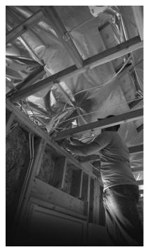
99% Aluminum-clad Mylar (rip-stop) White Color (one-side)
